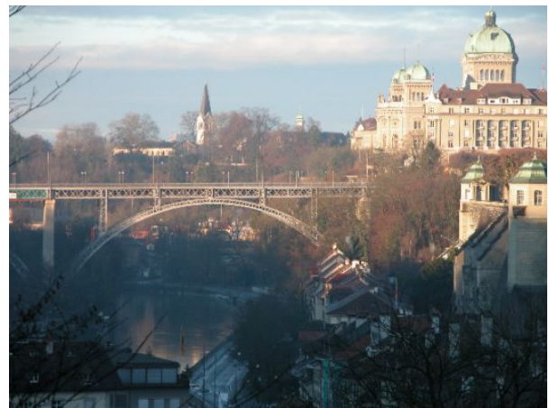
Figure 6: The landmark steel bridge in Bern to be instrumented with Sensima Inspection SHMEC crack monitoring technology.
